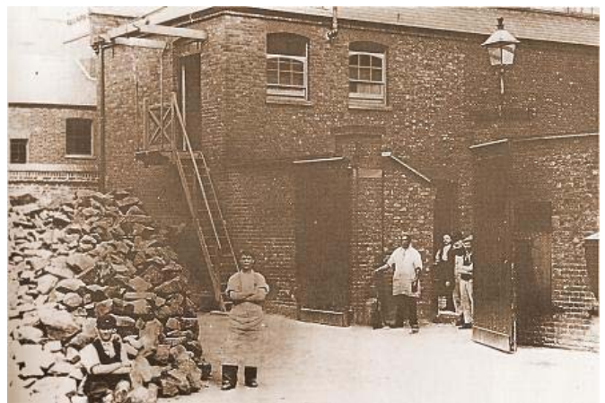
Stone Yard at the Hackney Union Workhouse
